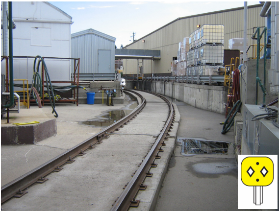
Restricted clearance in a customer siding Inset: Restricted clearance sign
