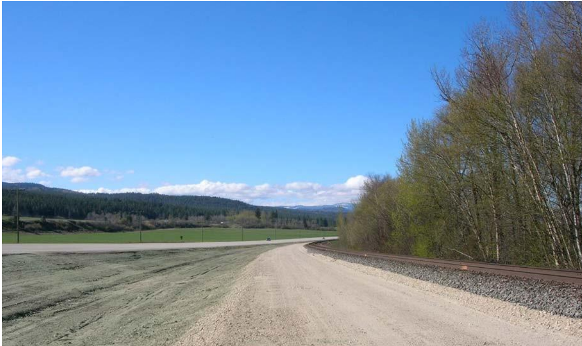
Figure 4: Seeding of Disturbed Areas
